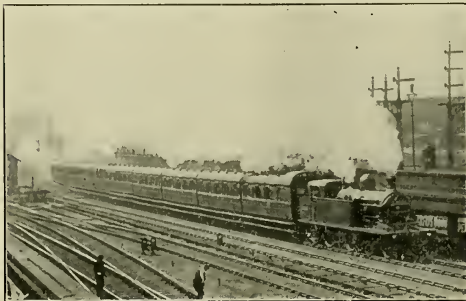
London & North Eastern Railway 10 Car Train With Vacuum Brake
